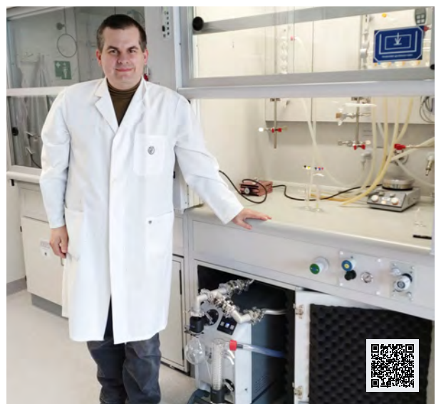
Network pump for two synthesis fume hoods at the Max Planck Institute
